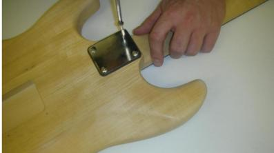
With the body placed on a protective surface face-up, position the neck into the neck pocket until fully inserted.
